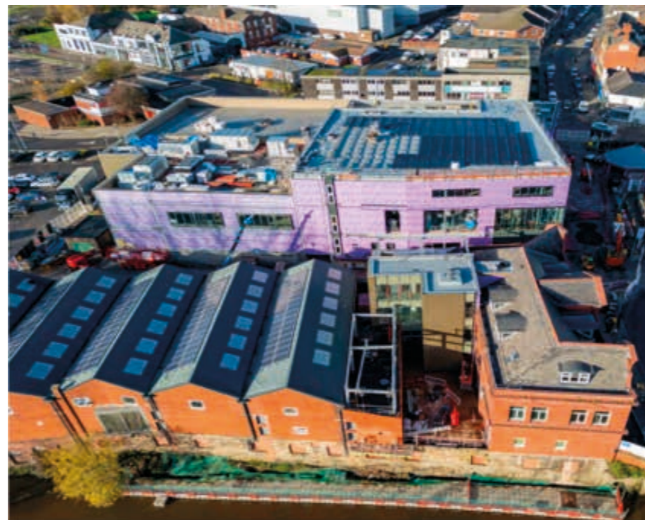
Radcliffe Hub (in construction)
