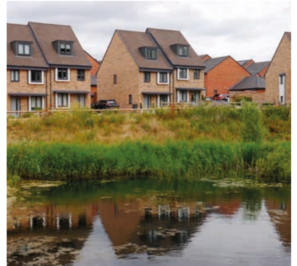
Example of drainage feature
