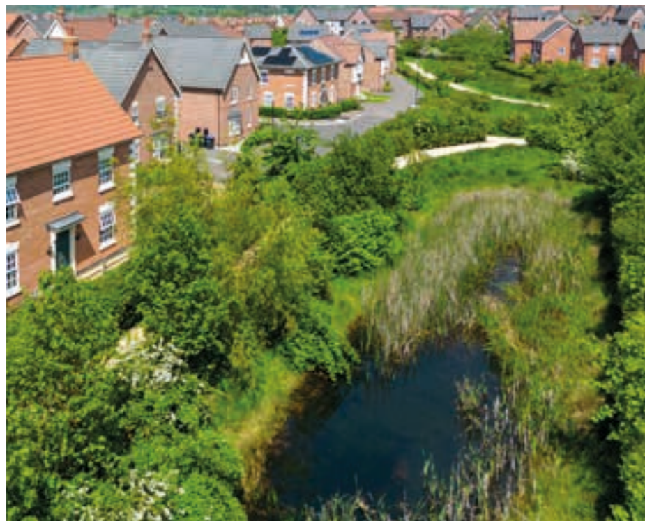
Example of drainage feature integrated within green corridor
